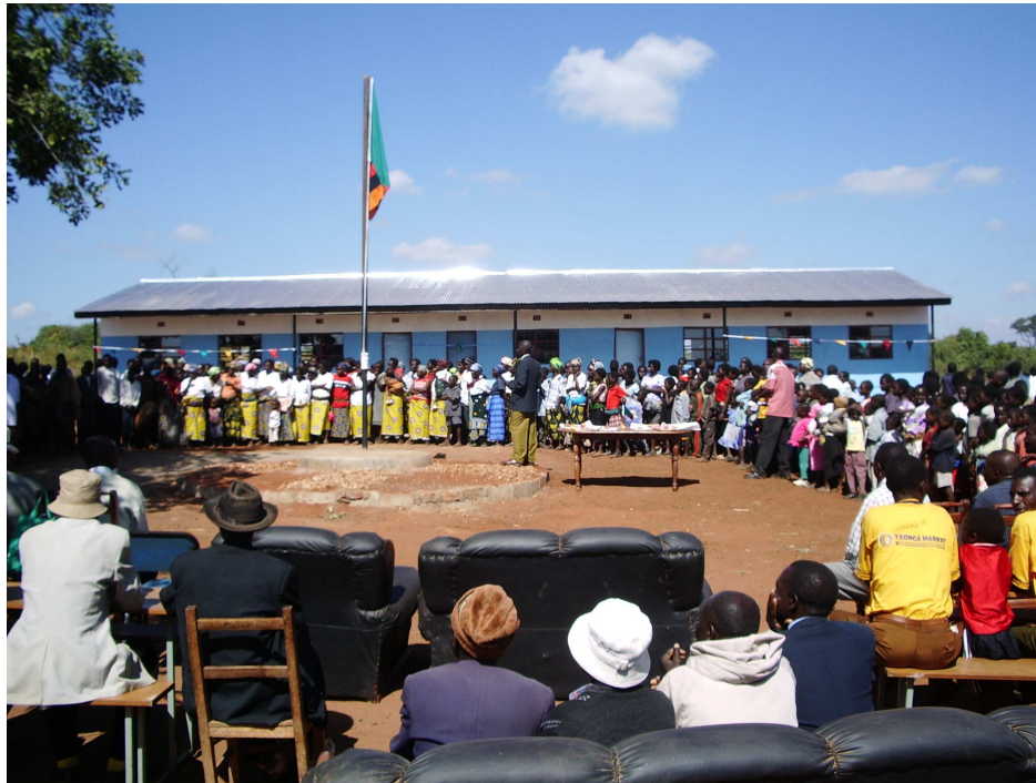
Opening of Nangombe school building, May 2006
